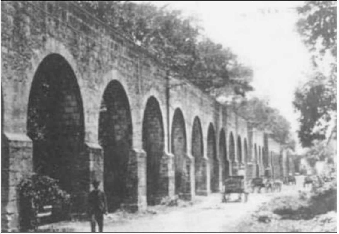
PHOTO 1 The aqueduct of Morelia in the early years of the twentieth century
