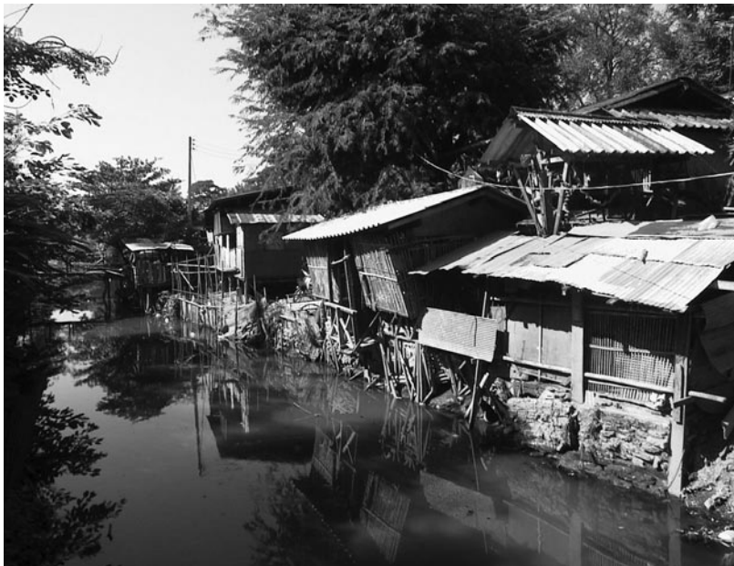
Photo 1: Constructions reach the Mae Kha canal embankments (photograph taken in November 2000)
