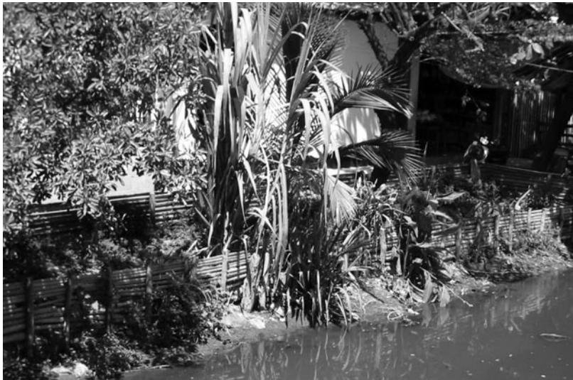
Photo 5: Eroded embankments on the Mae Kha canal have been restored by residents a number of times. This photograph shows the use of plants and bamboo fences to protect the embankment from erosion (photo taken in February 2003)
