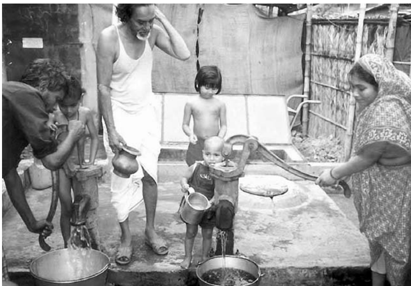
Photo 1: Water points consist of an underground storage reservoir, two hand-operated pumps and space for bathing and laundry
