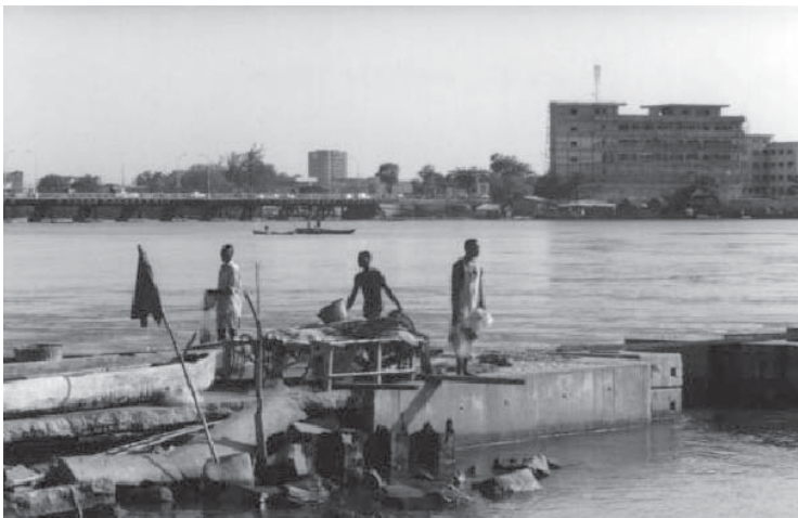
PHOTO 5 The concrete barrier on which fishermen stand at the entrance to Cotonou Lagoon
