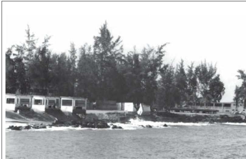
PHOTO 1 Hotel infrastructure (holiday village) being destroyed by coastal erosion
