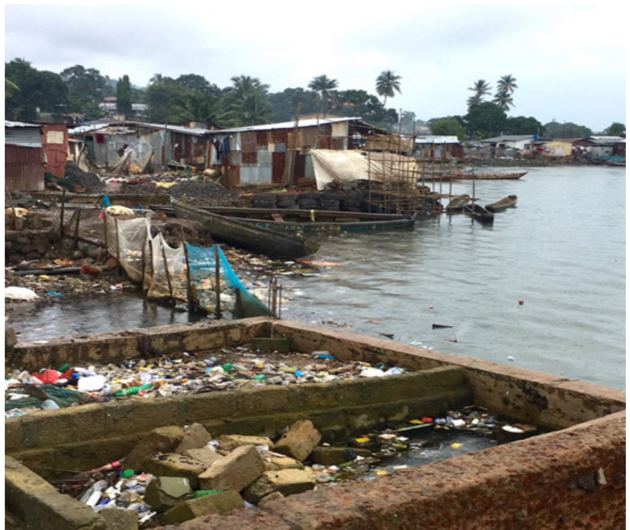
Settlement on a flood-prone area. Photo credit: A Allen (2016).
