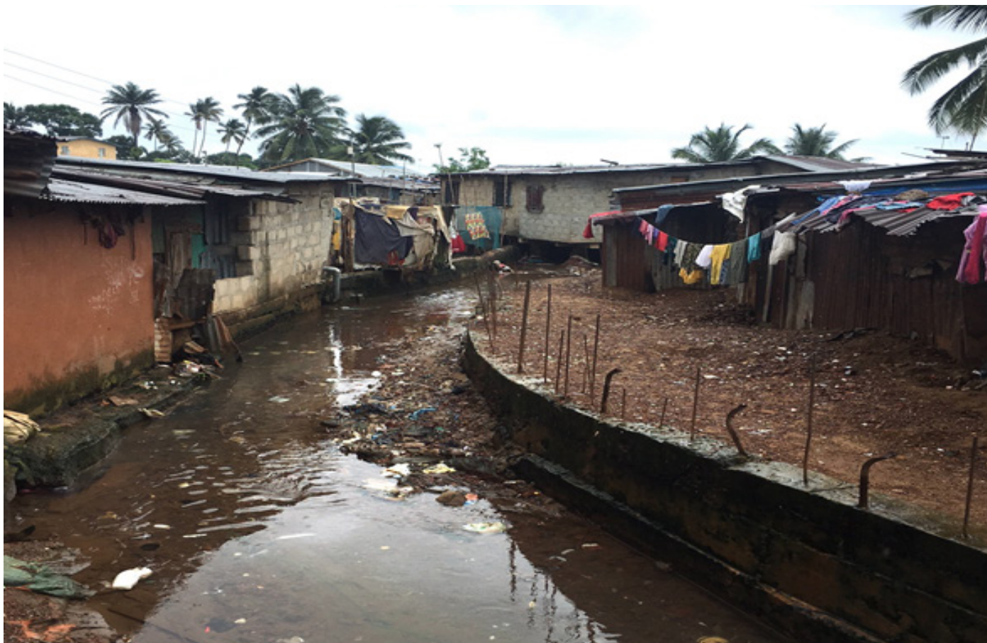
Large open drain running through the settlement in Cackle Bay, Freetown (Photo E. Osuteye, 2016).
