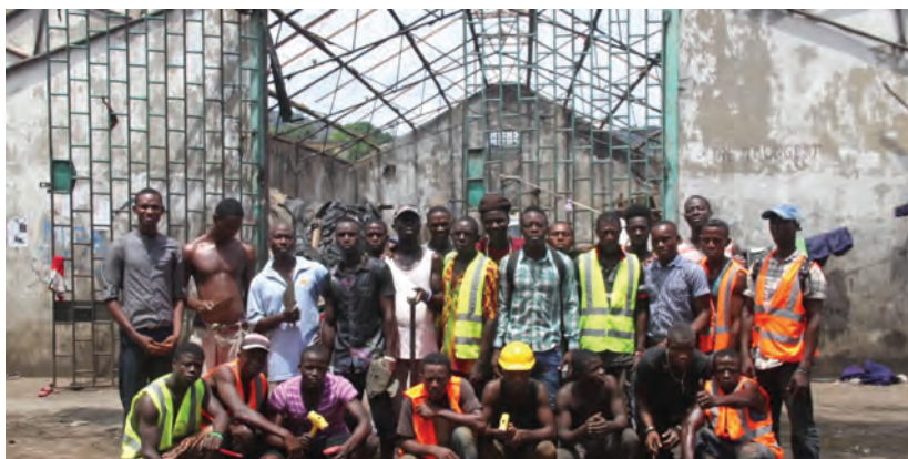
Photo 10: Le Plastics working on a new warehouse in Kingtom landfill site. (Le Plastics, 2018)
