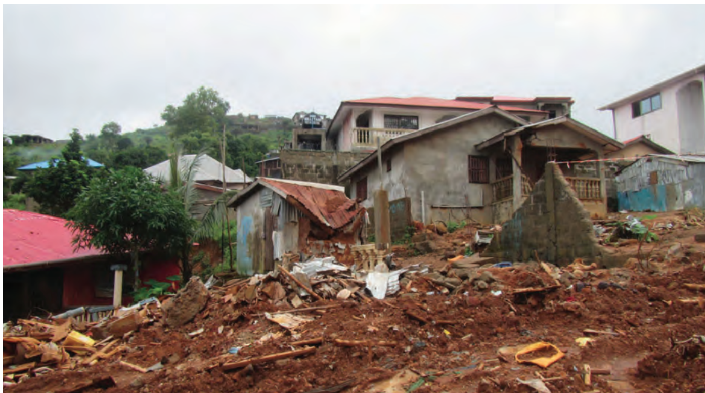
Landslide and Building Collapse. Photo Credit: World Bank Assessment on Landslides and Floods in the Western Area, 2017.
