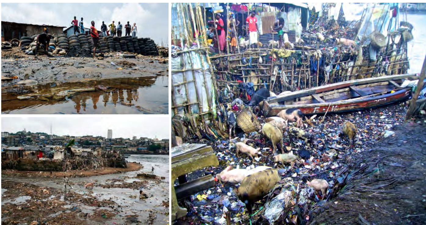
Top left: Banking with compacted mud in tires, Cockle Bay. Photo Credit: Nam Vo Son Bottom left: Banking with mud and waste in Susan's Bay. Photo Credit: Holly Pickett Right: Accumulated waste for later use in banking in Susan's Bay. Photo Credit Costa Anastasakis
