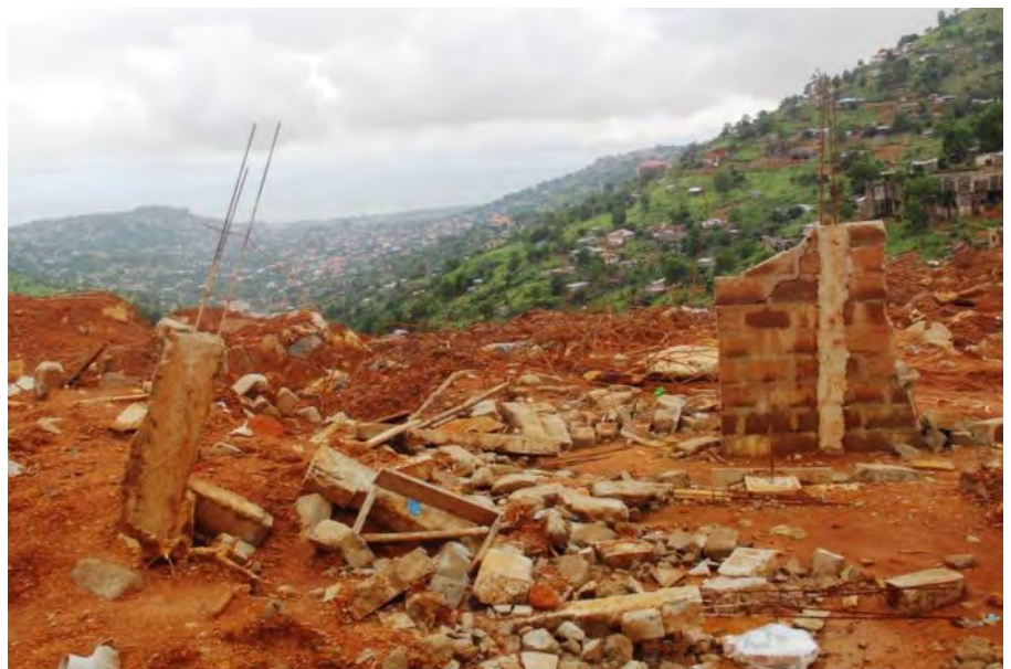
Fig 1: The ruins of buildings from the aftermaths of the mudslide in the Regent area, on the slopes of Sugarloaf Mountain Freetown, Sierra Leone, September 21, 2017. Photo Credit: Thomson Reuters Foundation / Eromo Egbejule.
