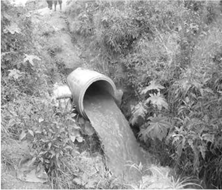
PHOTO 1 Culvert in the middle of the dam wall
