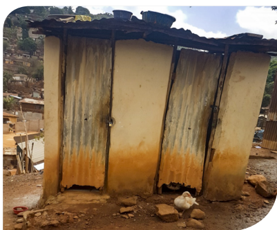
Photos of a pit toilet (left) and a hanging toilet (right)
