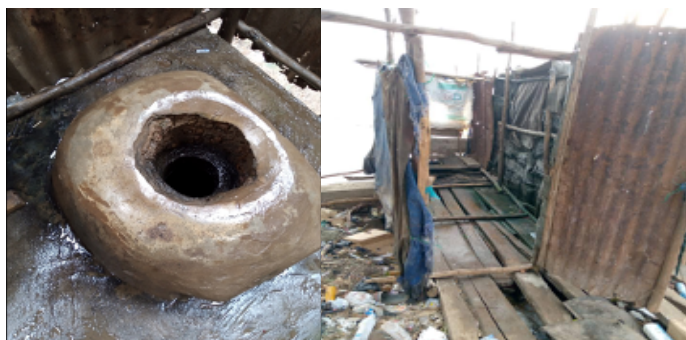
Figure 5: Unimproved toilet facilities in Portee-Rokupa. Left: A pit latrine. Right: A Hanging toilet. Photo credit: Amadu Labor, SLURC.
