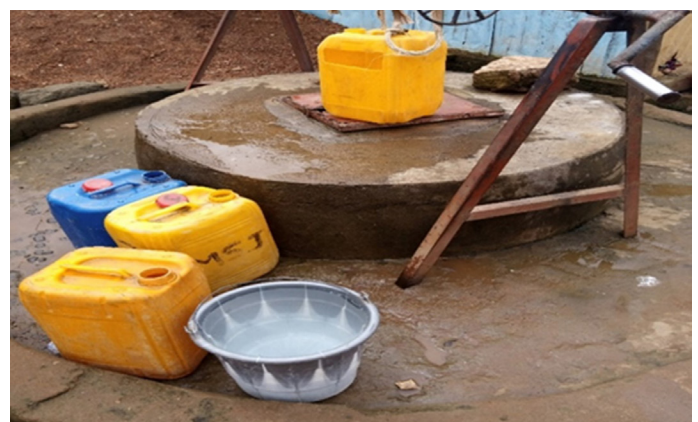
Figure7: Protected well at Portee-Rokupa. Photo credit: Amadu Labor, SLURC.
