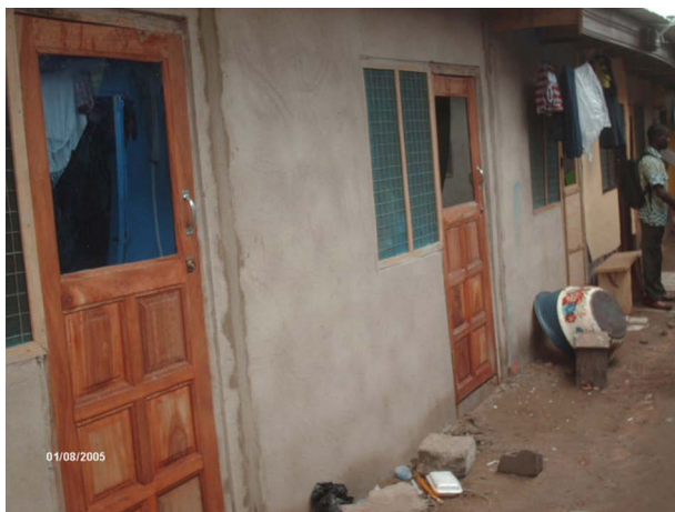
PHOTO 4 A newly constructed structure following the fire outbreak
