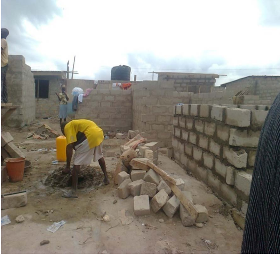
PHOTO 3 Community members' efforts to erect concrete structures after the incident
